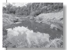
**EAST END SPOILS EXCAVATION:** Every year we dig out the large pond that we utilize to collect the silt that we pump out of the lake. It comes into the pond through a large pipe powered by the dredge, and then over the dredging season and afterward, the silt settles to the bottom. Then we hire a company to come in with an excavator to dig out the silt so that we can haul it away. This project has been completed and we estimate that 130 truckloads of dirt are
